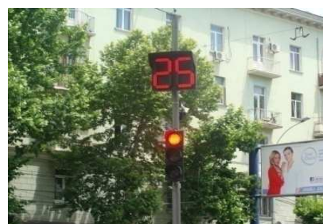
Picture 3: Traffic lights System in Tbilisi City
